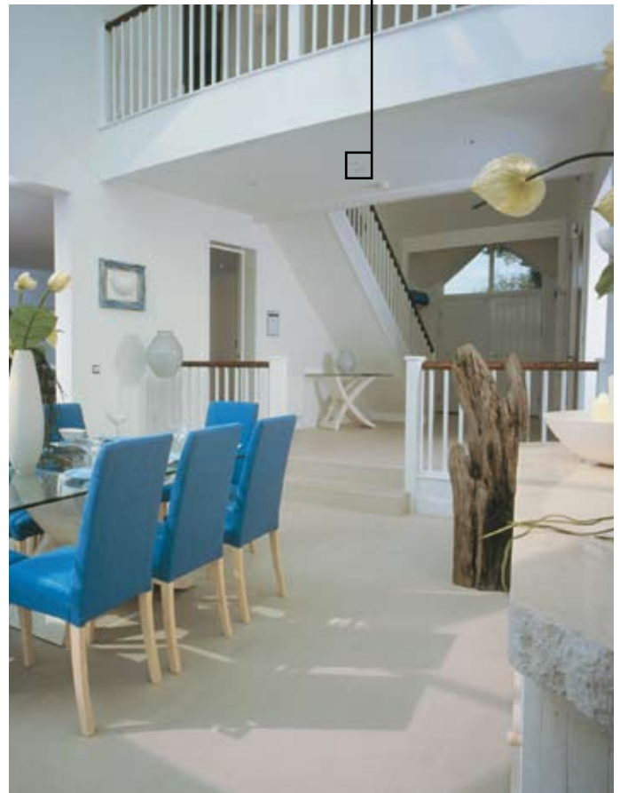
Unobtrusive sprinkler cover plate
