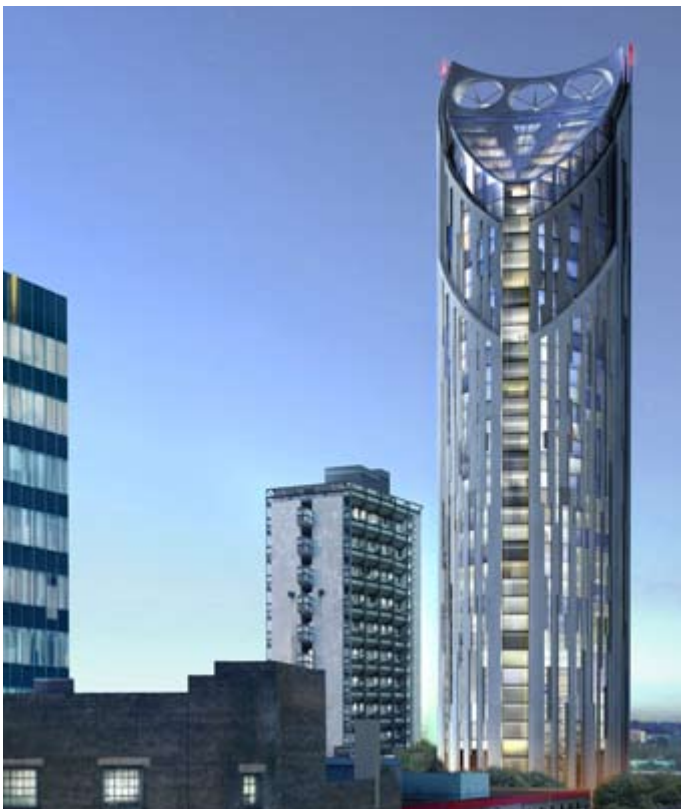
Greenflow favoured in fire engineered scenarios, due to additional reliability
